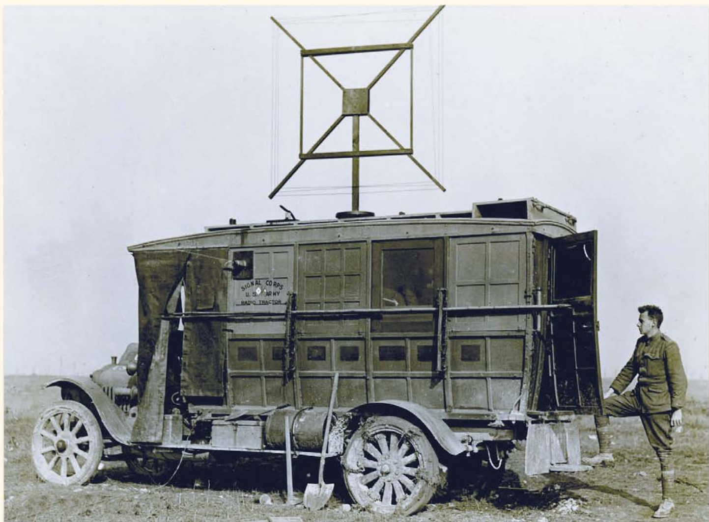
Below: the US Signal Corps apparently liked the White TBC and have fitted this one out as a 'Radio tractor'. (Photo NARA).
